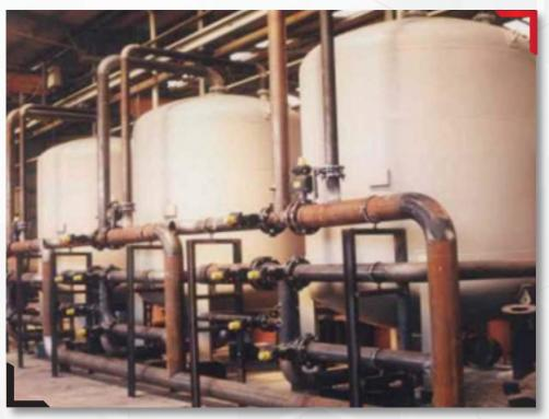
Capacity: 90 M3/H, Inside and Outside Sandblasting + Epoxy Coating, Full Automatic. Complete Weight: 24 Tons.
