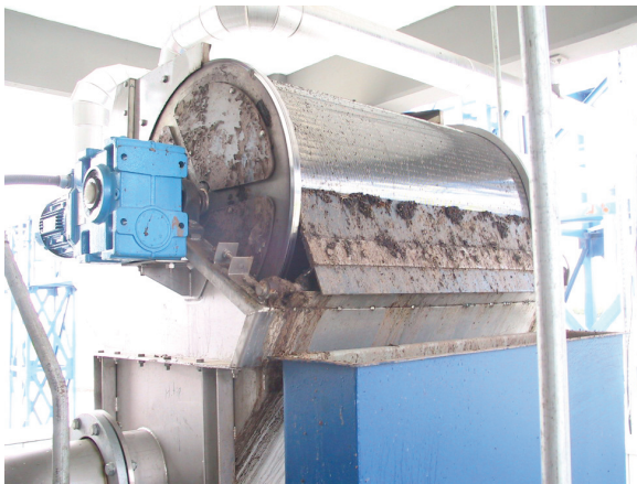
Rotating Drum Screen in operation
