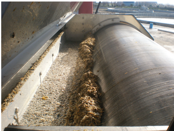
Detail showing feeding of the drum
