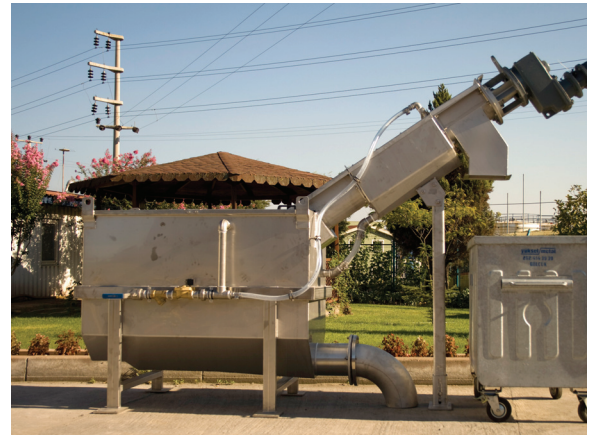
Sewage Acceptance Plant - SAP
