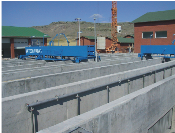
Installation of Travelling Grit Scrapers for twin tanks
