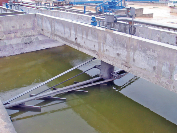
Central Driven Grit Scraper during installation
