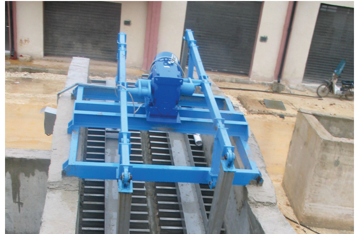
Double Degritter during installation
