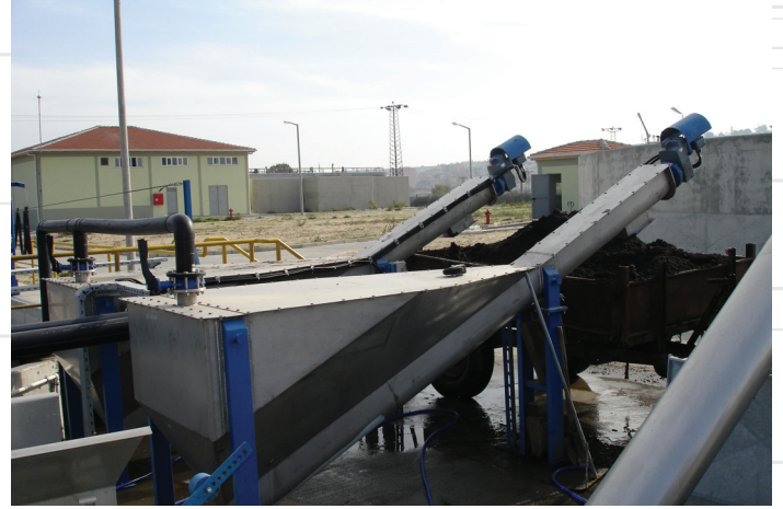
Grit Separators with inclined shaftless spiral
