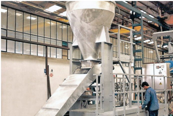
Grit Cyclone with Travelling Grit Scraper Bridge
