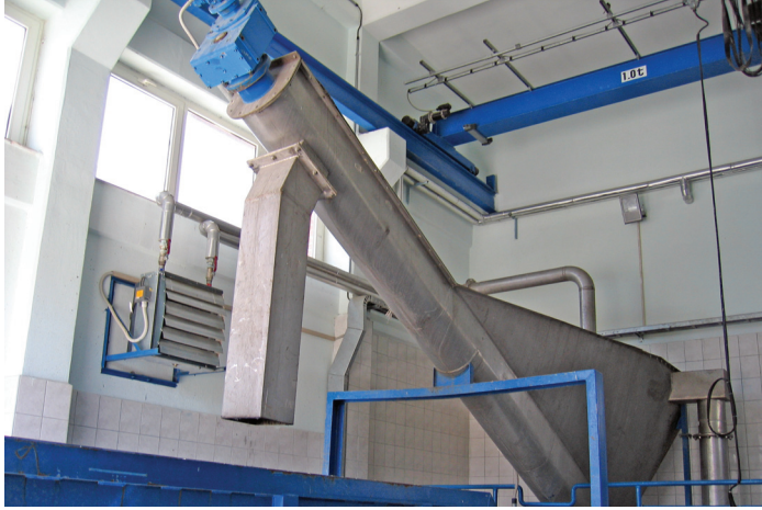
Grit Separator during operation
