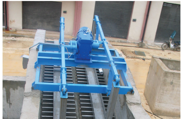
Double Degritter during installation
