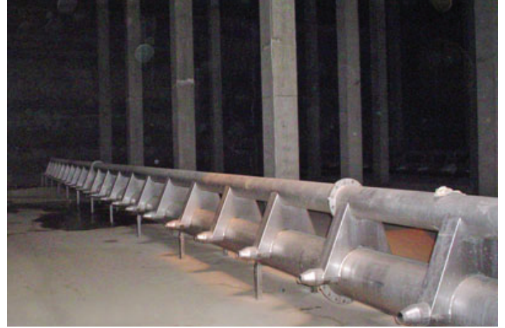
Jet Nozzle Aerators during installation
