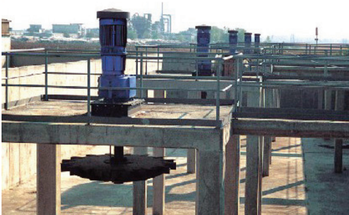
Installation of fixed type Vertical Shaft Turbine Aerators
