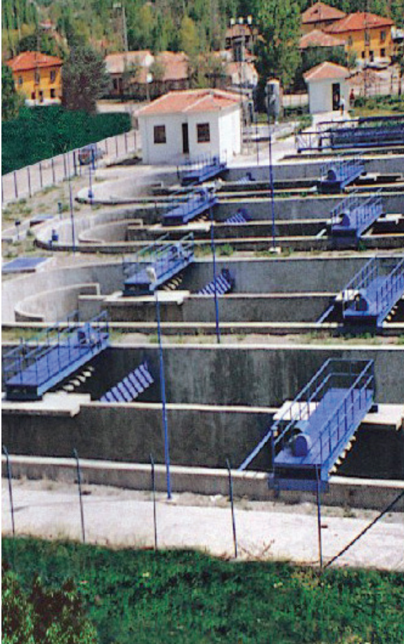
Horizontal Brush Aerators during installation
