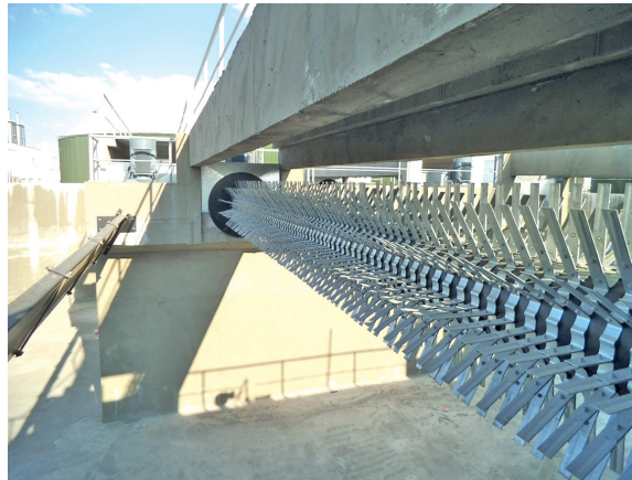
Blades, installed in a screw pattern prevents vibration
