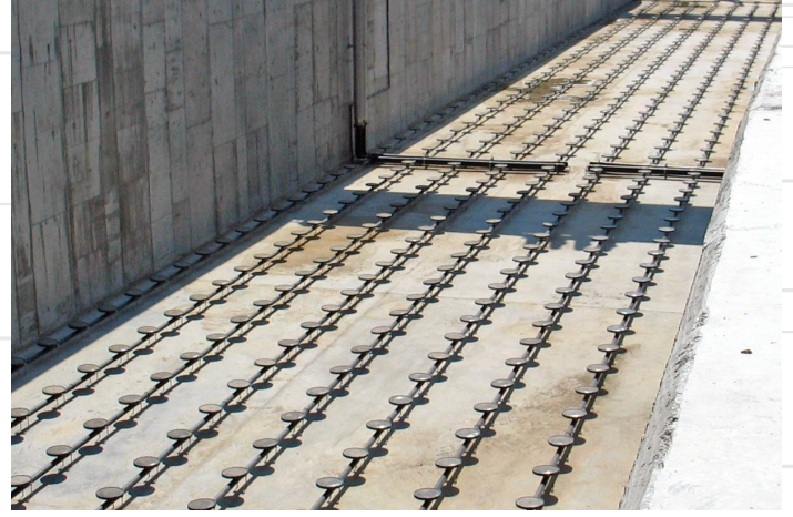
Installation of Diffuser Type Aeration System
