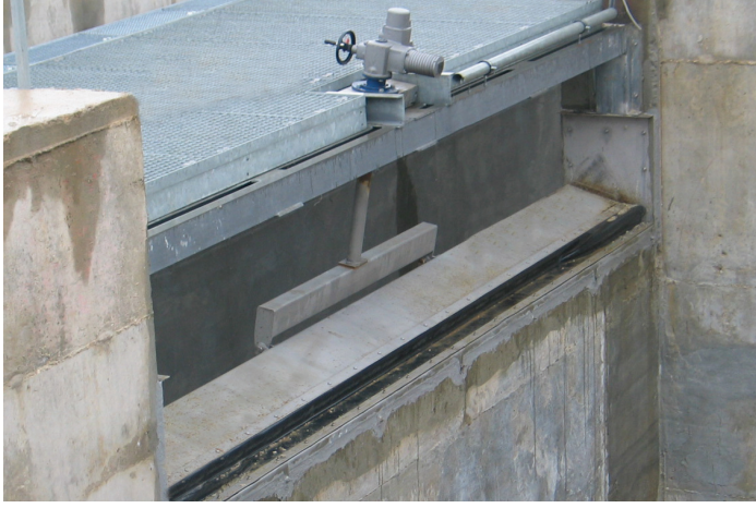
Motorized Adjustable Overflow Weir
