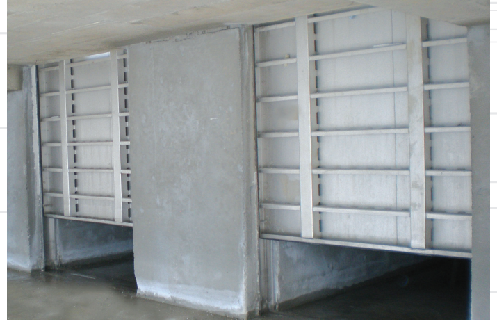
Penstocks closing the channels
