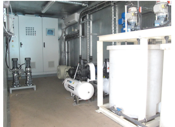
Internal view from a Control room
