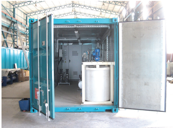
Control room inside a standard container
